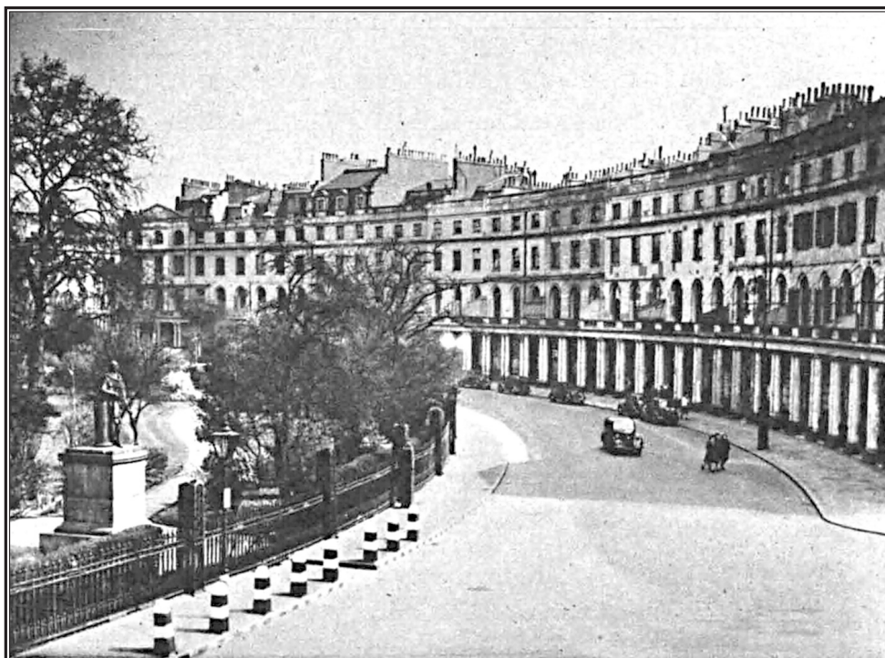
PARK CRESCENT, REGENT'S PARK: WHERE THE REPORT RECOMMENDS PRESERVING THE FAÇADE AND MAKING GOOD ANY GAPS CAUSED BY BOMBING,
