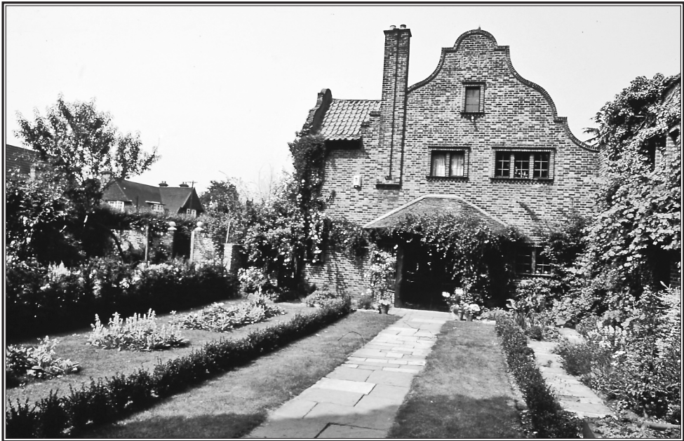
34. Greystones, Merton Park before restoration October 1991 (COURTESY CHRISTOPHER SPENCER)
