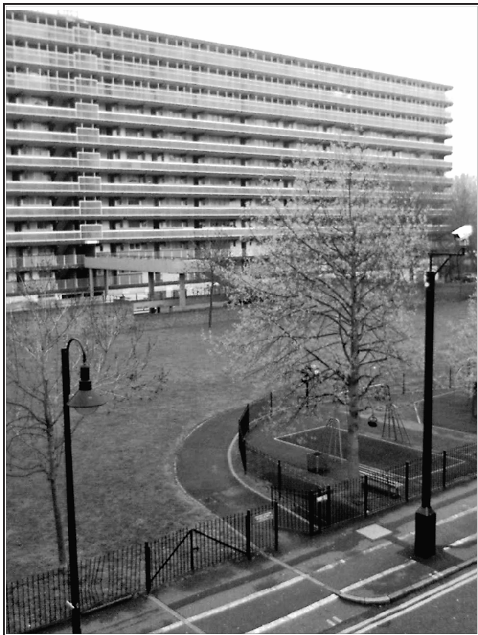
32. Photograph showing the grassed gardens at the foot of the Heygate Estate (COPYRIGHT MIKEY TOMKINS)
