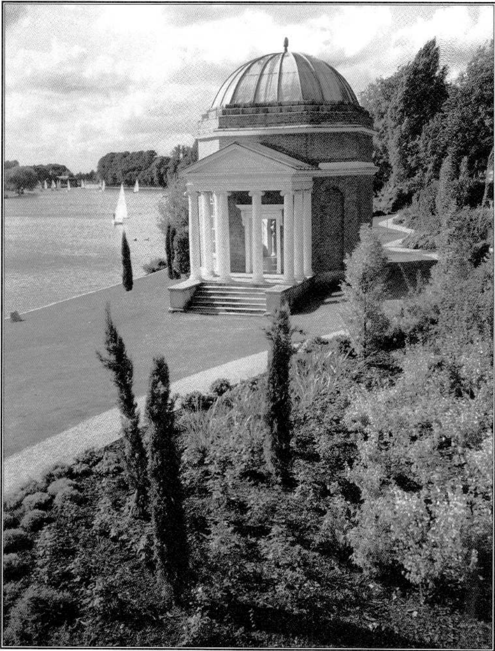
32. Garrick's Temple following restoration, 2000.
