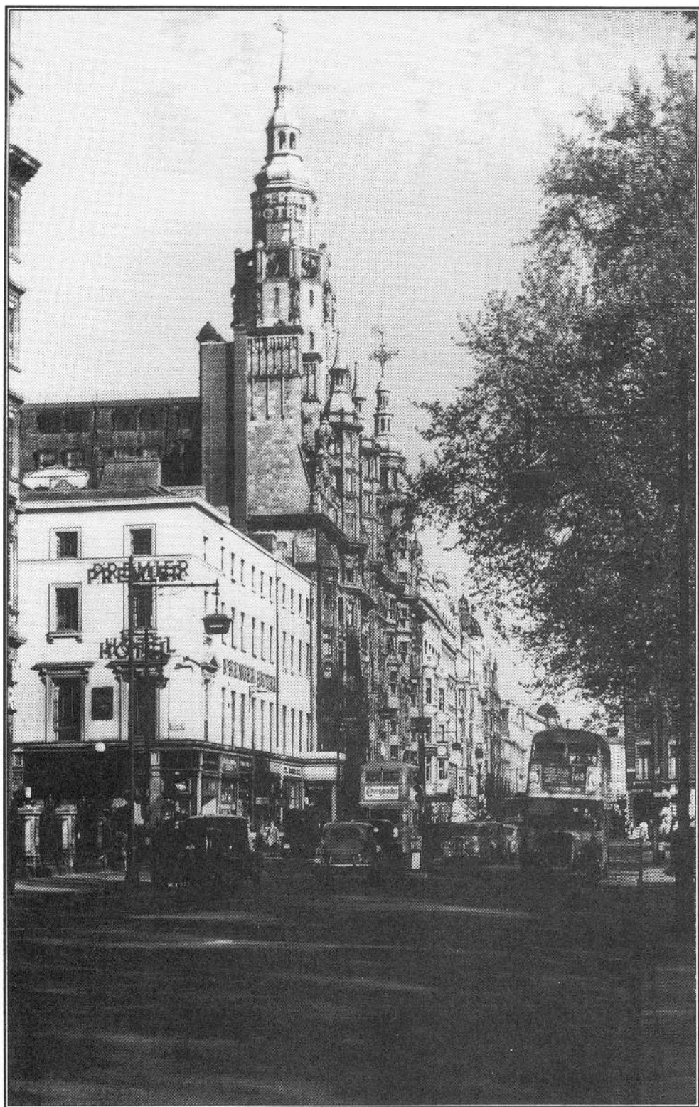
4. Russell Square as seen from Southampton Row, looking south towards the former Imperial Hotel, 1959. (LONDON METROPOLITAN ARCHIVES)
